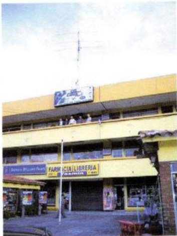
Antenna at TG0AA club station 009
